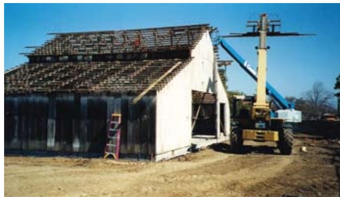
Disassembling the Bianchi barn for relocation.
